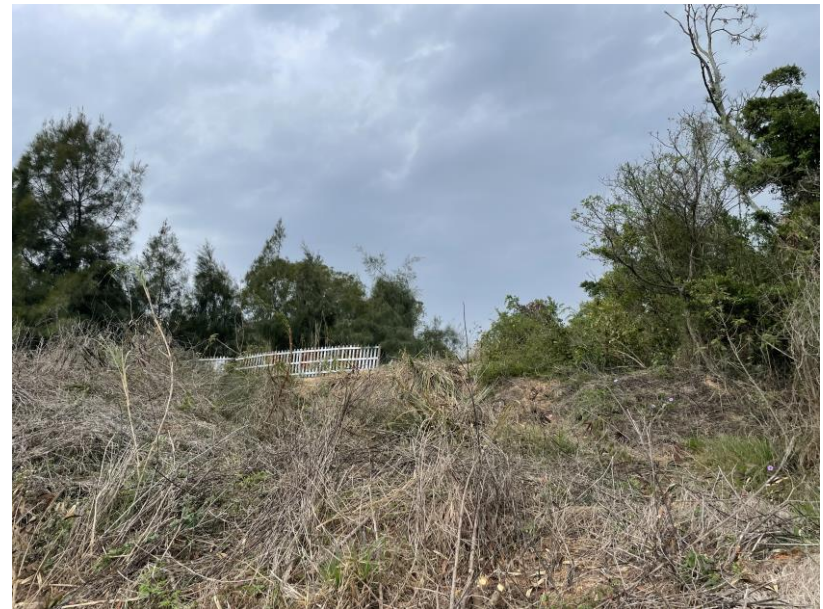
昔果山環場道旁圍籬損壞 (改善前)圖-2
